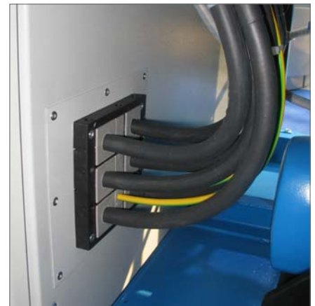
KEL 24|12-2MT - Page 22 Routing of 6 large cables up to 34 mm with one cable entry frame and one cut-out.
